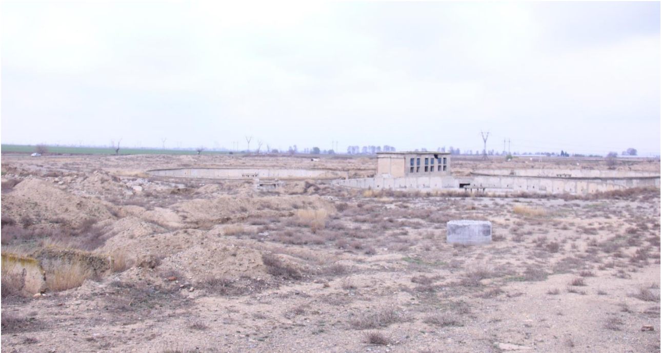
Figure 11. Unfinished oxidation pools of the original uncompleted WWTP
