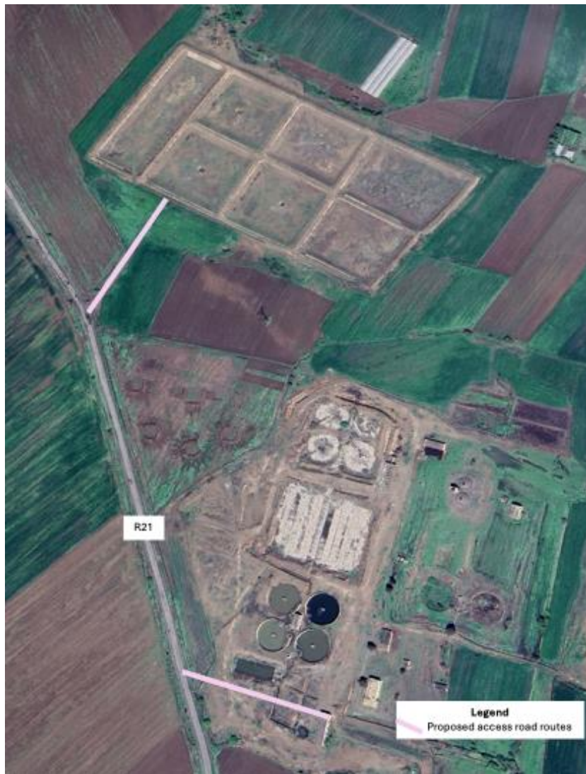
Figure 5. Proposed access road routes off the R21 to the WWTP site layout 18
